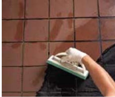
Figure 9.23 – Spreading of epoxy grout.
