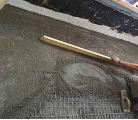
Figure 9.13 – Tile mechanic screeding a mortar bed.
