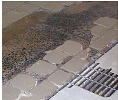
Figure 9.20 — Effects of inappropriate grout used on a demanding application. Notice not only the erosion of the grout joints, but also the adhesive mortar under the tile. In many floor applications, the use of an epoxy based adhesive and grout are required in order to ensure long-term performance.
