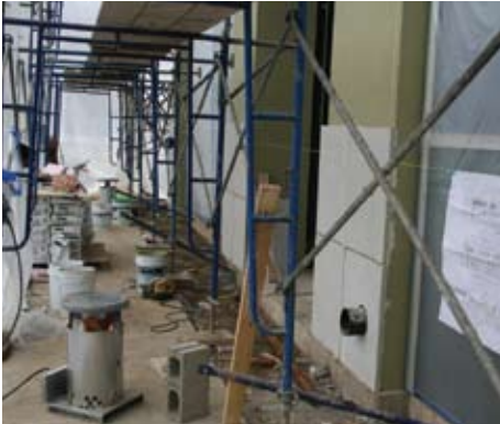
Figure 10.1 — Exterior façade work in temporarily heated, tented area in the middle of winter. LATICRETE Headquarters building, Bethany, CT in January 2008.
