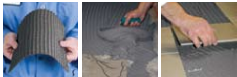
Figure 8.1 — Trowel applied sound and crack adhesive mortar applied to concrete substrate.
