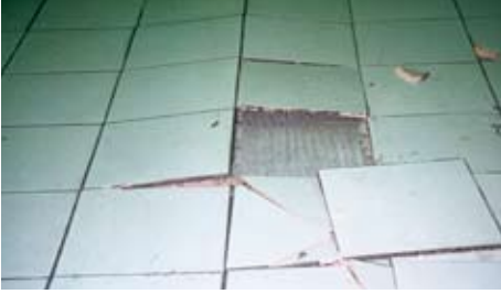
Figure 4.4 – Result of stresses induced by concrete shrinkage and lack of movement joint control. As the concrete shrinks, expansion joints are required to relieve the stress. When expansion joints are omitted or are not sufficient, “tenting” of the tiles can occur, creating bond failure and cracking.
