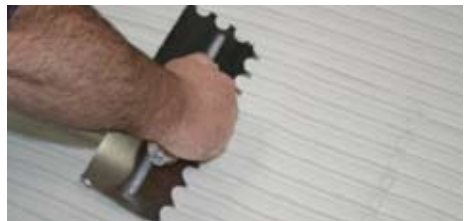
Figure 9.5 – Trowel applied medium bed mortar with a 3/4" (19mm) loop notch trowel used for large format tiles or stones. Trowel medium bed mortar in one direction holding trowel at a 45 degree angle. Notice the full ribbons of mortar that are left behind.
