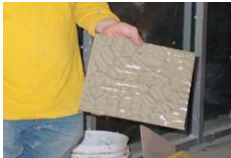
Figure 9.9 — Ceramic tile removed during the installation to verify proper coverage is being attained. Notice the lower right hand corner of the tile is lacking coverage. This could well lead to a cracked tile.
