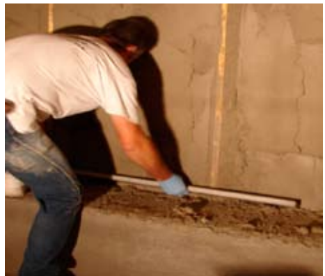
Figure 9.15 – Latex fortified render is being applied to wall surface. Notice the lath strips that are set into the mortar. The lath strips are leveled and plumbed to establish the correct wall render depth. Once the render achieves a sufficient cure, the lath strips are carefully removed and the cavities are filled with mortar.
