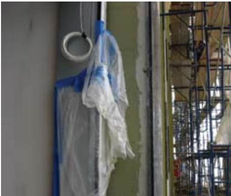
Figure 10.2 – Example of tubular scaffolding with weather protection enclosing the building.
