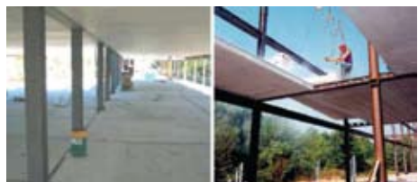
Figure 4.27 — Pre Cast Concrete Planks. Planks rest and are supported by a flange attached to the steel girders. The planks are hoisted into place by a crane and mortared to the beams and to each other. Photo courtesy of Girder Slab Technologies LLC.
