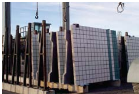
Figure 7.12 – The panels are ready to be loaded and transported to the project site.
