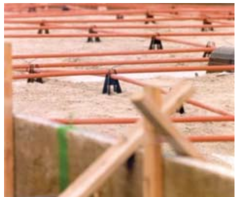
Figure 4.25 — Post Tensioned Concrete Cables — Notice the Orange Tensioning Cables That Will Run Throughout the Concrete Slab — Photo Courtesy of SunCoast Post Tensioning Company.
