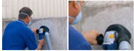
Figure 4.7 – Dustless Grinding.
