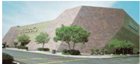
Figure 9.1 — High adhesive shear and tensile strength to resist seismic movement. Before photograph of the Bullock's building prior to the Northridge, CA earthquake in 1994. Tiles were installed on the exterior façade with LATICRETE® 4237 Latex Additive mixed with LATICRETE 211 Powder over LATICRETE 9235 Waterproofing Membrane.
