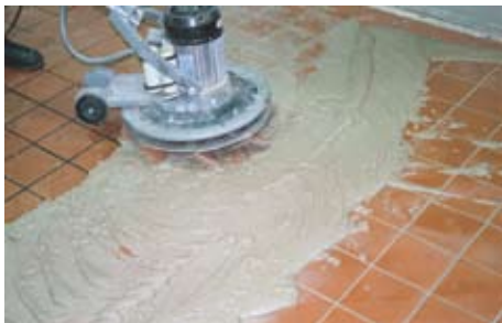
Figure 10.26 — Grout Spreading Process.
