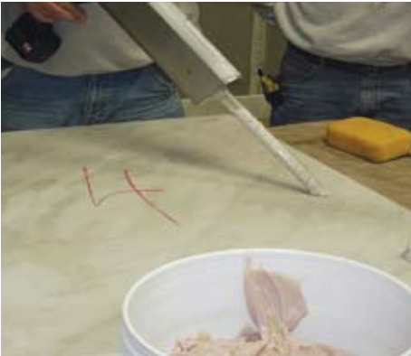
Figure 9.17 — Epoxy spot bond (e.g. LATAPOXY® 310 Stone Adhesive) adhesive is applied to the back of the stones with an automated epoxy mixer / applicator. A minimum of 10% adhesive coverage is generally required. The LATAPOXY 310 Stone Adhesive is available in standard grade (maximum working time of 45 minutes) or rapid grade (maximum working time of approximately 5 minutes).
