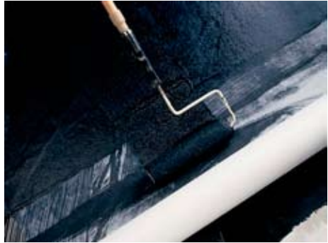
Figure 8.2 — Liquid applied membrane applied to concrete substrate.
