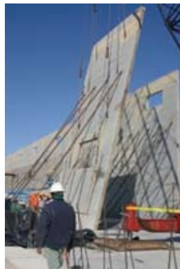
Figure 5.1 — Tilt Up Concrete Panels erected into place. Photo courtesy of www.constructionphotographs.com .
