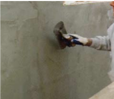
Figure 9.14 – Tile mechanic applying latex fortified cement based scratch coat to a block wall with a hawk and trowel.
