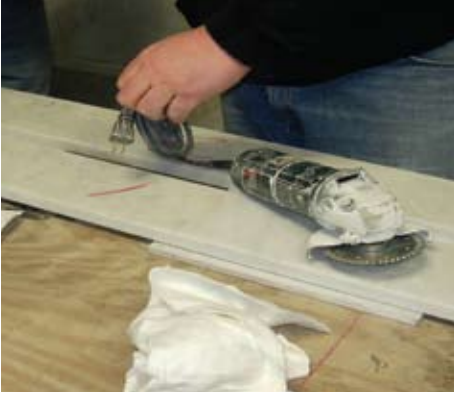
Figure 9.16 — Stone is prepared for installation by the epoxy spot bond method. Stone back is roughened at the adhesive connection points then washed and allowed to dry.
