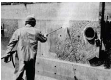
Figure 5.2 — High-Pressure Water Washing.
