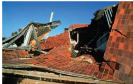
Figure 9.2 — High adhesive shear and tensile strength to resist seismic movement. Photograph of the Bullock's building after the Northridge, CA earthquake in 1994. Tiles remain adhered after severe shear stress from seismic activity and structural failure.
