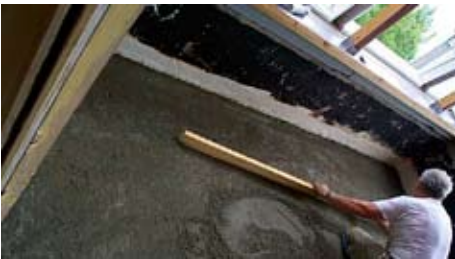
Figure 4.10 – Installation of an unbonded wire reinforced mortar bed.
