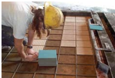
Figure 7.8 – Negative Cast Method. Tiles are pressed finish face down into molds. Notice the key backed (dove tails) configuration of the tiles.
