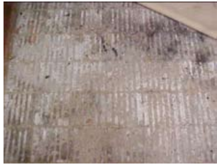
Figure 4.23 – Presence of Efflorescence on surface of concrete slab. Moisture migration through the slab can carry destructive salts to the surface of the concrete slab.
