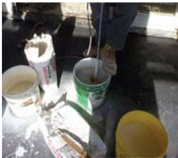
Figure 9.3 – Mixing of liquid latex fortified portland cement medium bed mortar.
