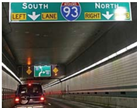
Figure 7.13 – Tiled pre-cast vertical panels (Ted Williams Tunnel, Boston, MA).
