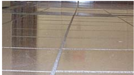
Figure 9.4 – Large format tile highlight imperfections in the substrate.
