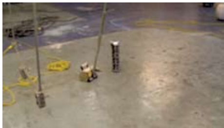
Figure 6.1 – Epoxy Painted / Coated Floor exhibiting wear in traffic areas due to heavy fork lift traffic and chemical attack. (Photo courtesy of Allied Maintenance Group, LLC).
