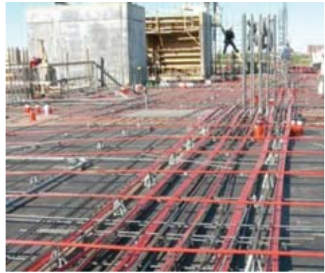
Fig. 4.24 — Post Tensioned Concrete Slab — Notice the Orange Tensioning Cables That Will Run Throughout the Concrete Slab — Photo Courtesy of SunCoast Post Tensioning Company.
