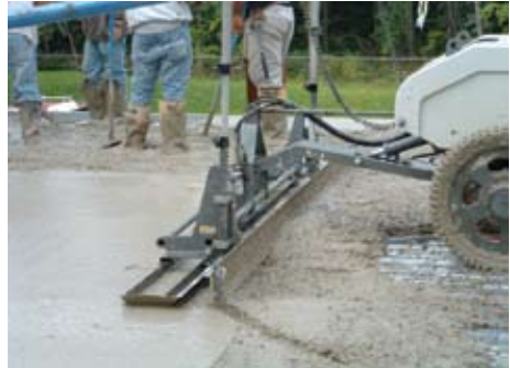
Figure 4.12 – Placement and screeding of elevated concrete slab over steel pan.
