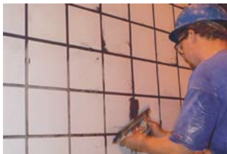
Figure 7.10 – Once the tiled panels are cured, the grouting process can begin. These panels are grouted with LATICRETE SpectraLOCK® PRO Grout®.
