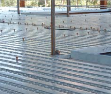
Figure 4.28 — Steel Pan Showing Placement of Shear Connections and Edge Detail.
